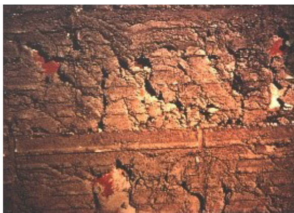
Photo 6 Poorly Filled Collar Joint
