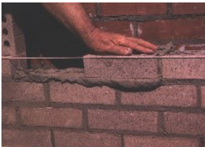
Photo 1 Shoving Brick into Place
