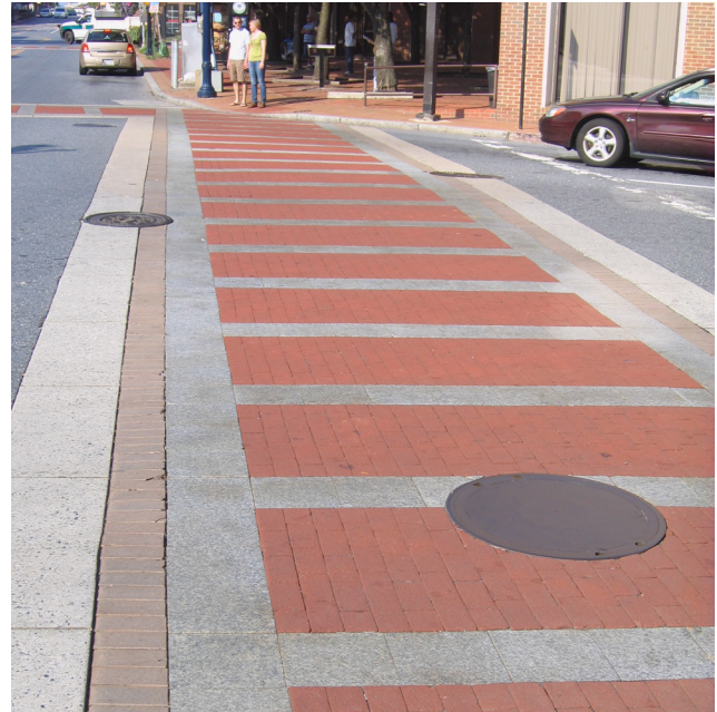
Photo 12 Smooth Transition for Utility Structure
