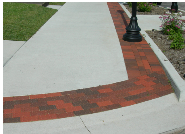
Photo 14 Curb Cut and Pavers with Detectable Warning Surfaces
